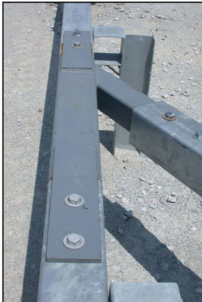
Figure 12. Y Splice Connection for BEAT-BP
