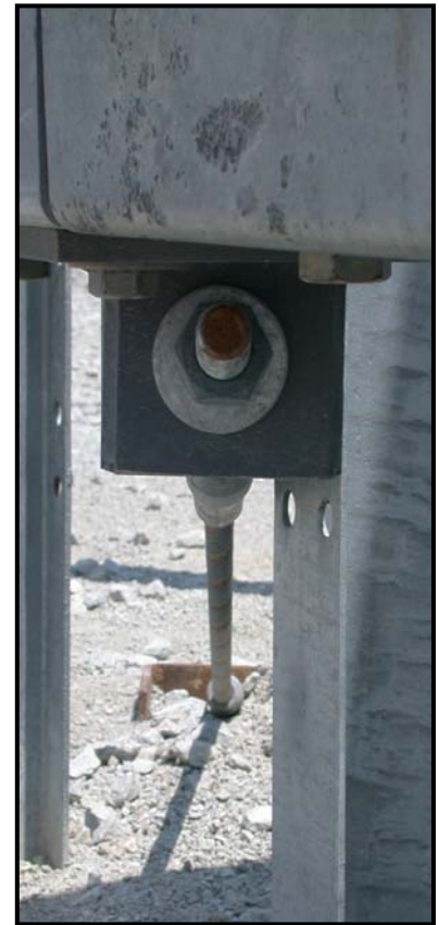
Figure 5. Interior Anchor Detail for the BEAT-BP
