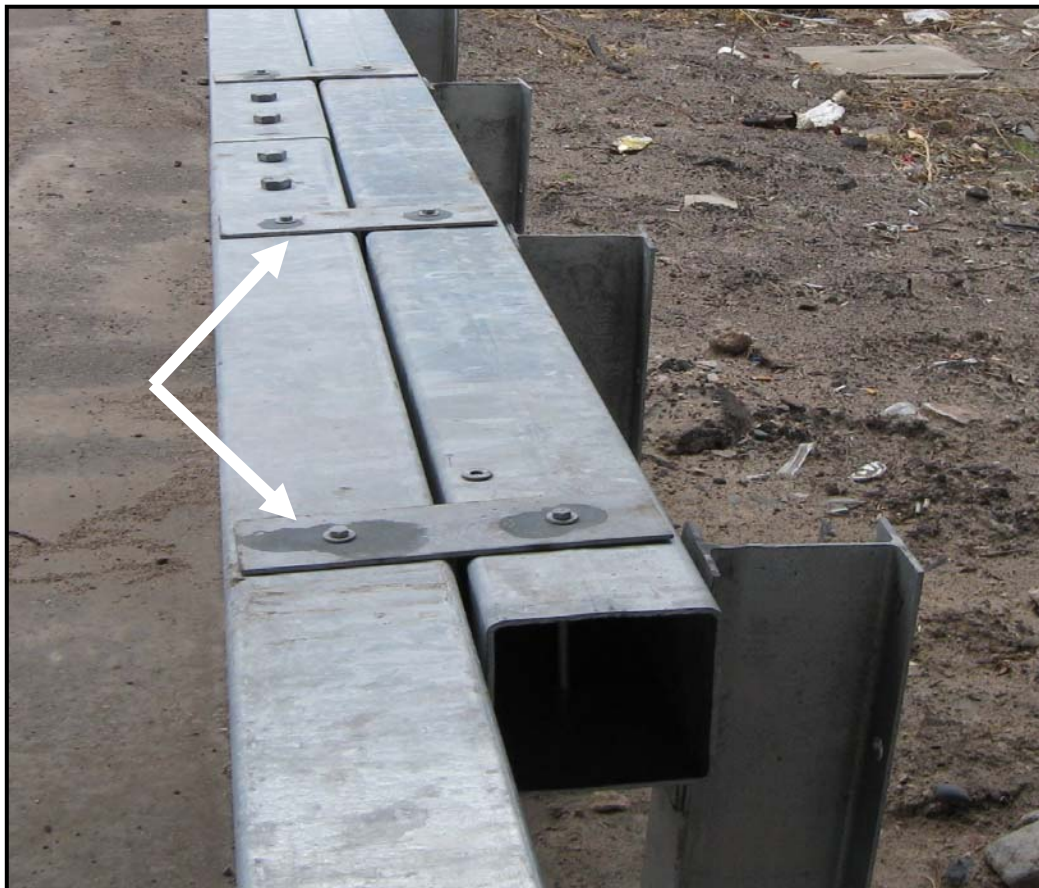
Figure 16. Tie Plate Connection for BEAT-BP
