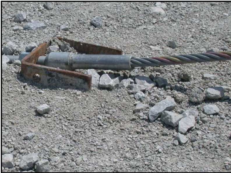
Figure 5. Interior Anchor Detail for the BEAT-BP
