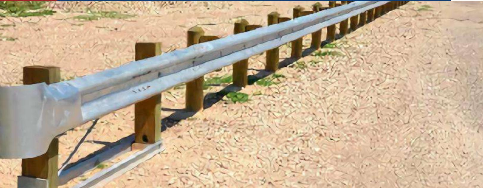
The Downstream Anchor Terminal (DAT) system is a non-proprietary design for anchoring 31" rail. It is not intended to be hit head on and therefore should only be used on the trailing end of a piece of guardrail.
