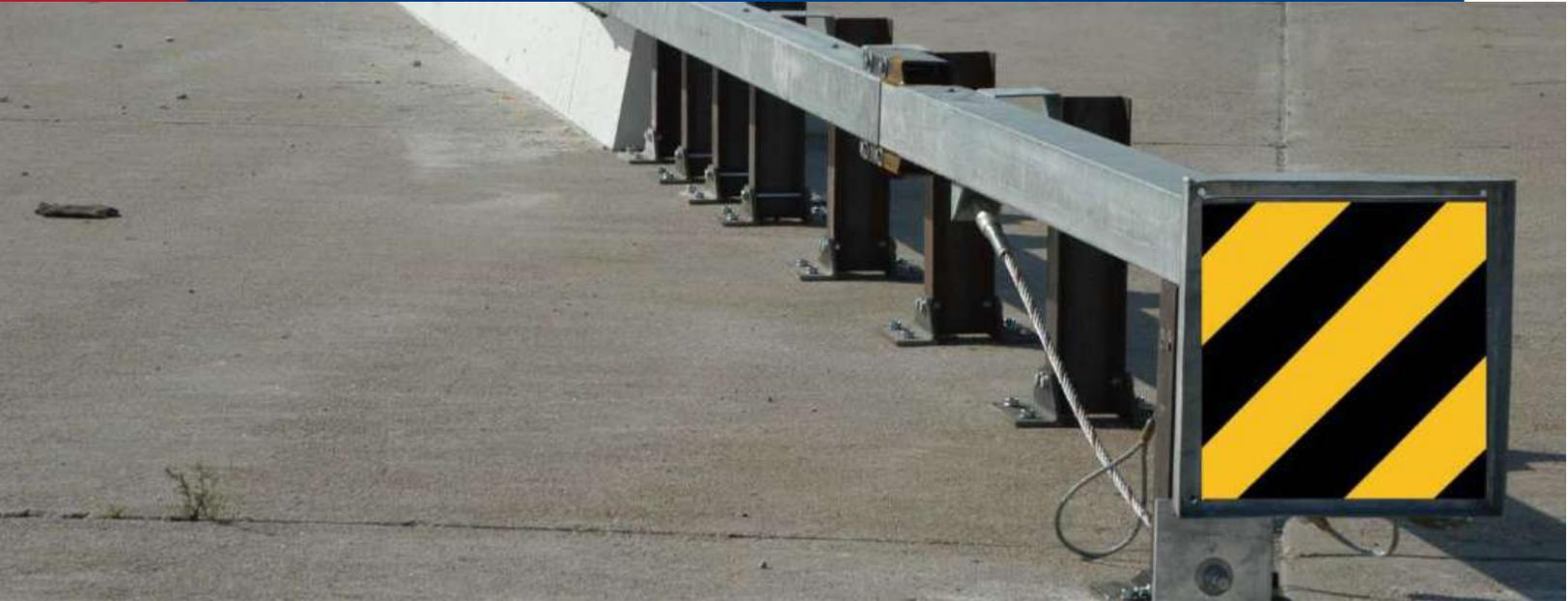
Box Beam Bursting Energy Absorbing Terminal – Single-Sided Crash Cushion The BEAT-SSCC offers a low cost option to protect the ends of rigid barriers. There is an option for driven ground mounted posts or surface mounted posts anchored to a concrete foundation. Variable lengths of 28', 32', 36', 40, 44' for sites needing additional length-of-need are available upon request.
