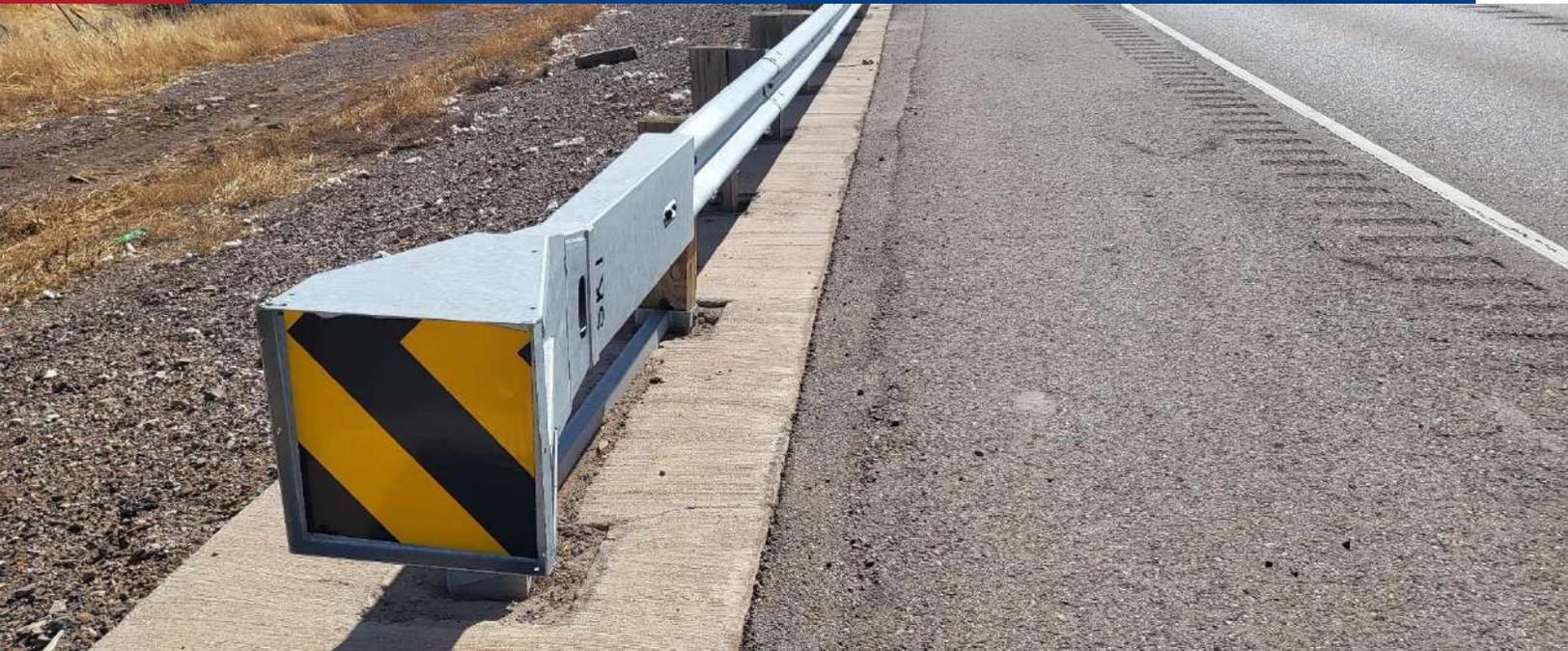
The SKT (Sequential Kinking Terminal) is an energy absorbing tangent terminal.
